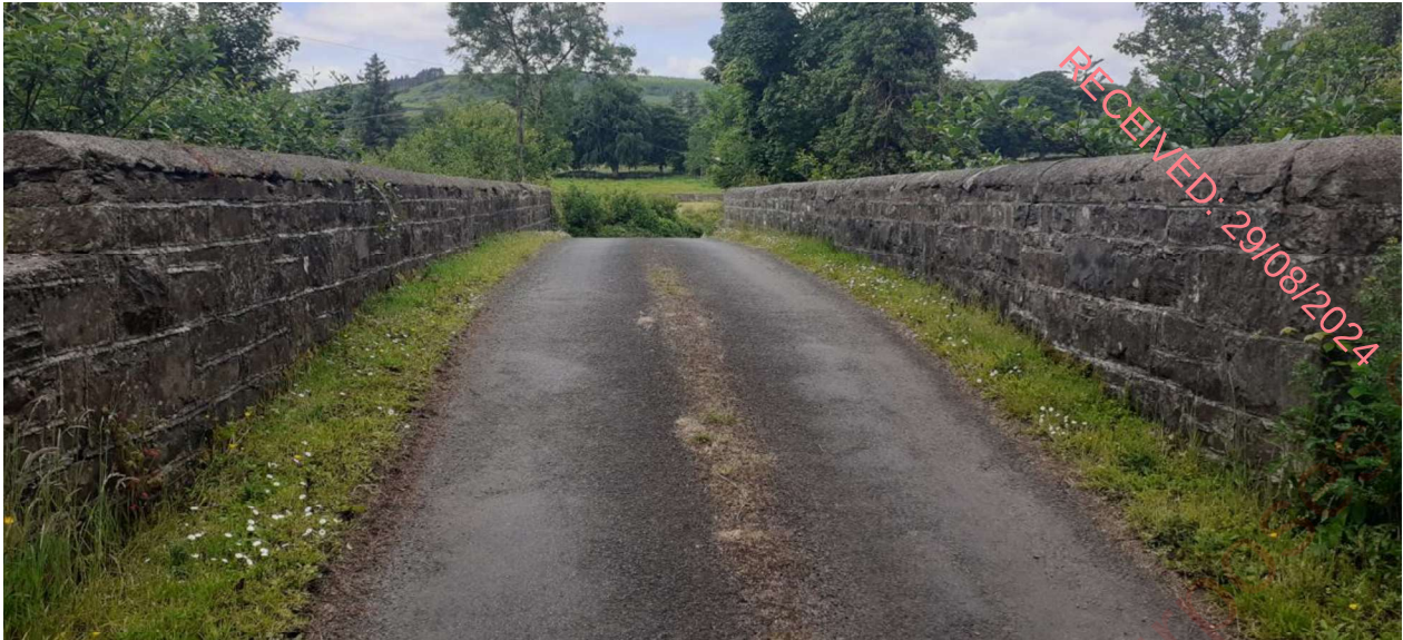
Figure 14.7 – 4m Wide Ballinglen River Bridge Note poor visibility of oncoming vehicles
