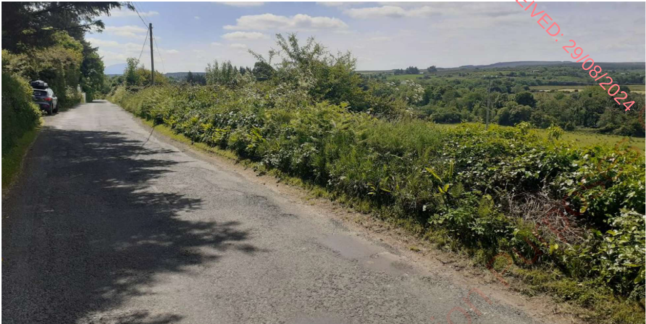
Figure 14.26: View South from R315 Centreline at Location of Proposed Temporary Access Junction Note no crest or sag in road prohibiting junction visibility if the boundary hedge is set back/ removed.
