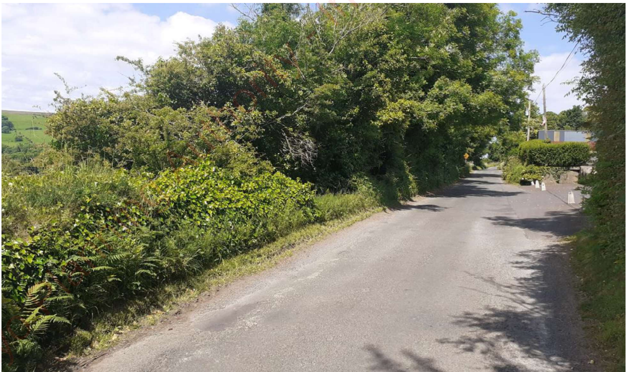
Figure 14.25: View North from R315 Centreline at Location of Proposed Temporary Access Junction Note no crest or sag in road prohibiting junction visibility.
