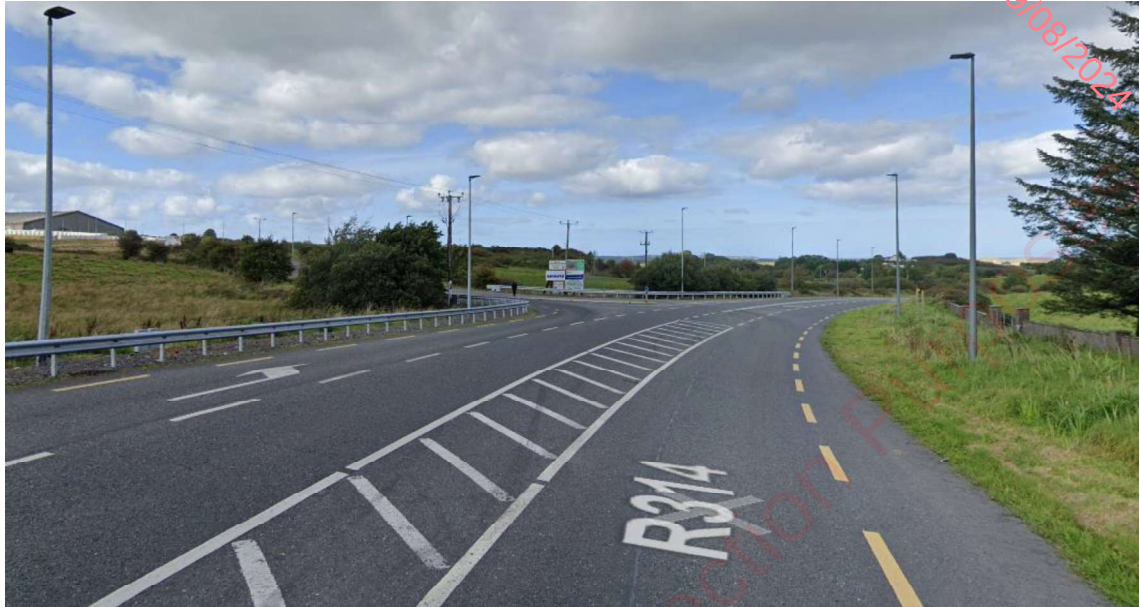
Figure 14.18: The Killala Business Park Access Junction
