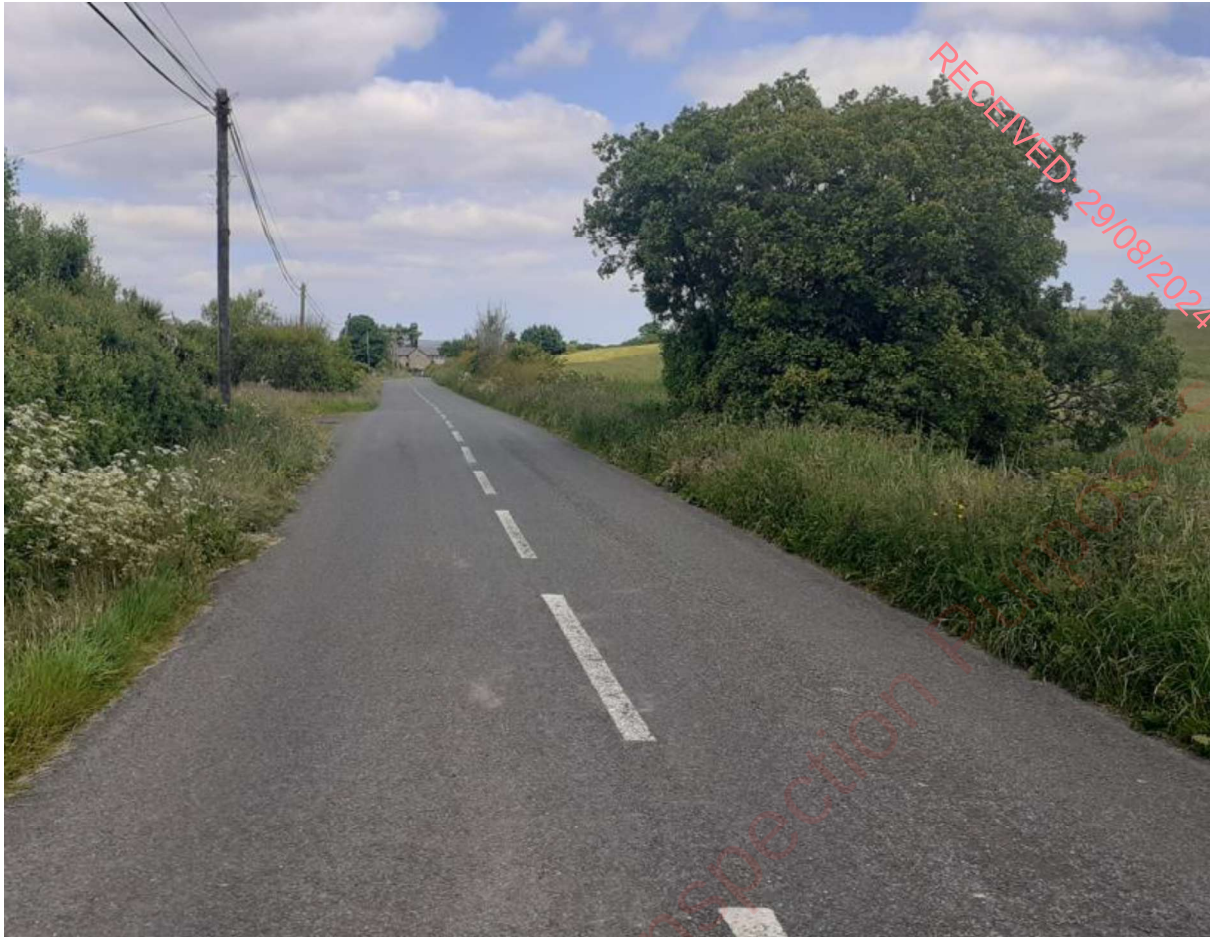
Figure 14.4: R315 - Typical Formation and Road Conditions
