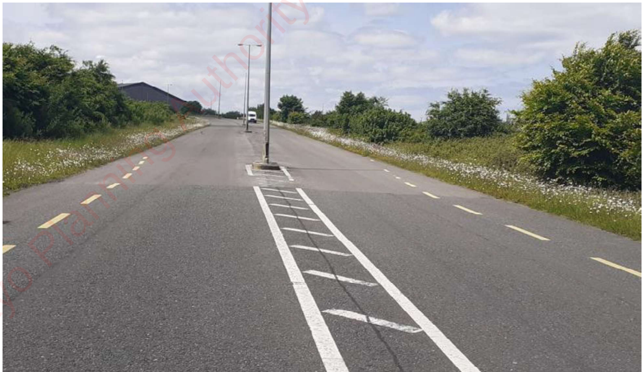
Figure 14.19: The Killala Business Park Access Road: Road Conditions and Formation
