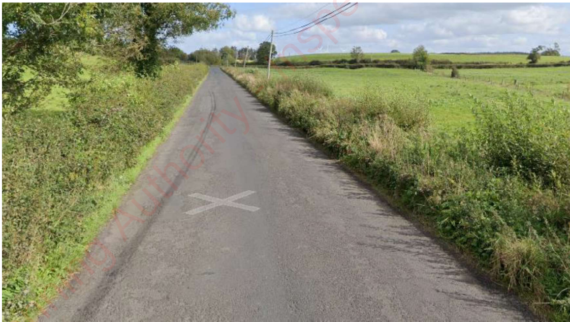
Figure 14.13: L1101 Local Road – Typical Road Conditions and Formation
