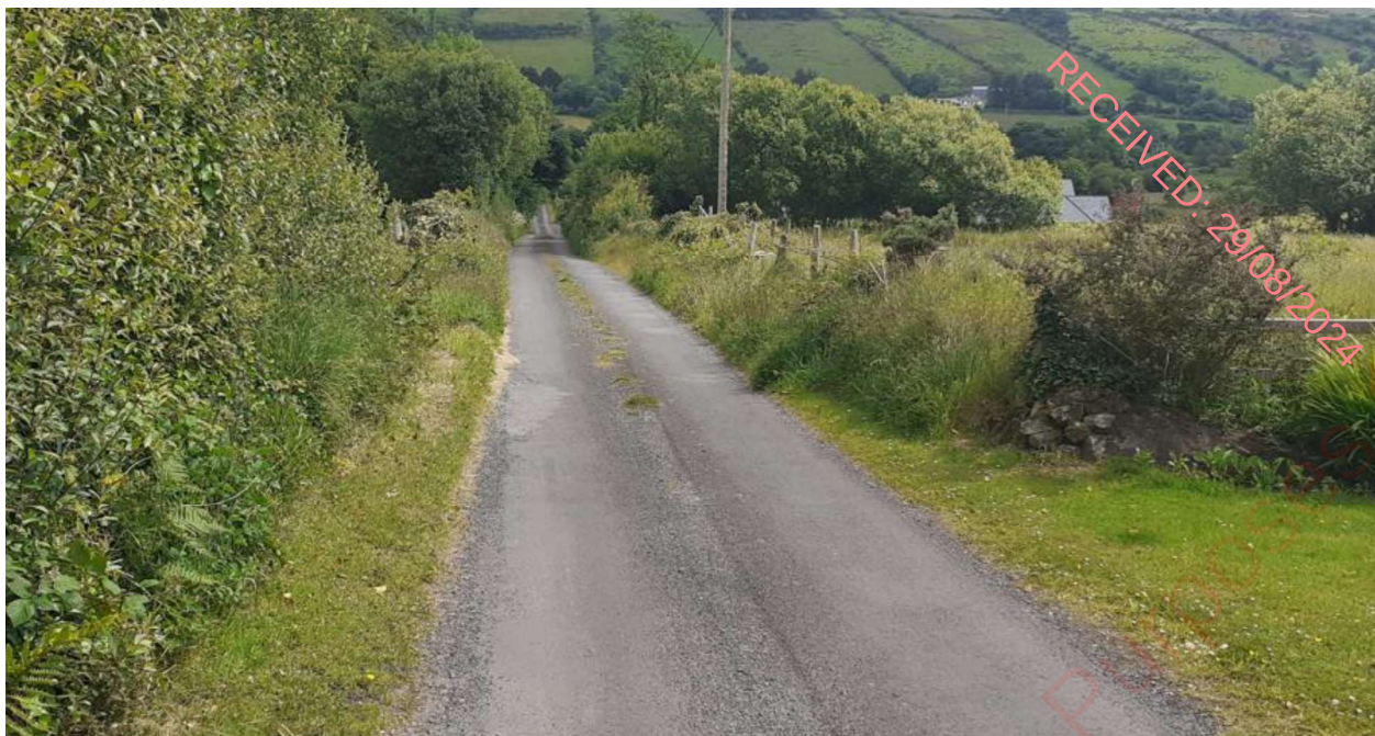
Figure 14.5: Local Access Road – Typical Road Conditions and Formation
