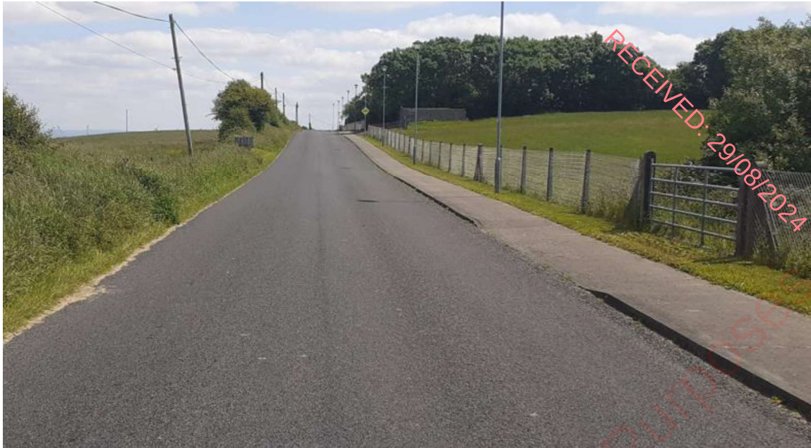
Figure 14.14: L11101 Local Road through Kincon – Typical Urban Road Conditions and Formation
